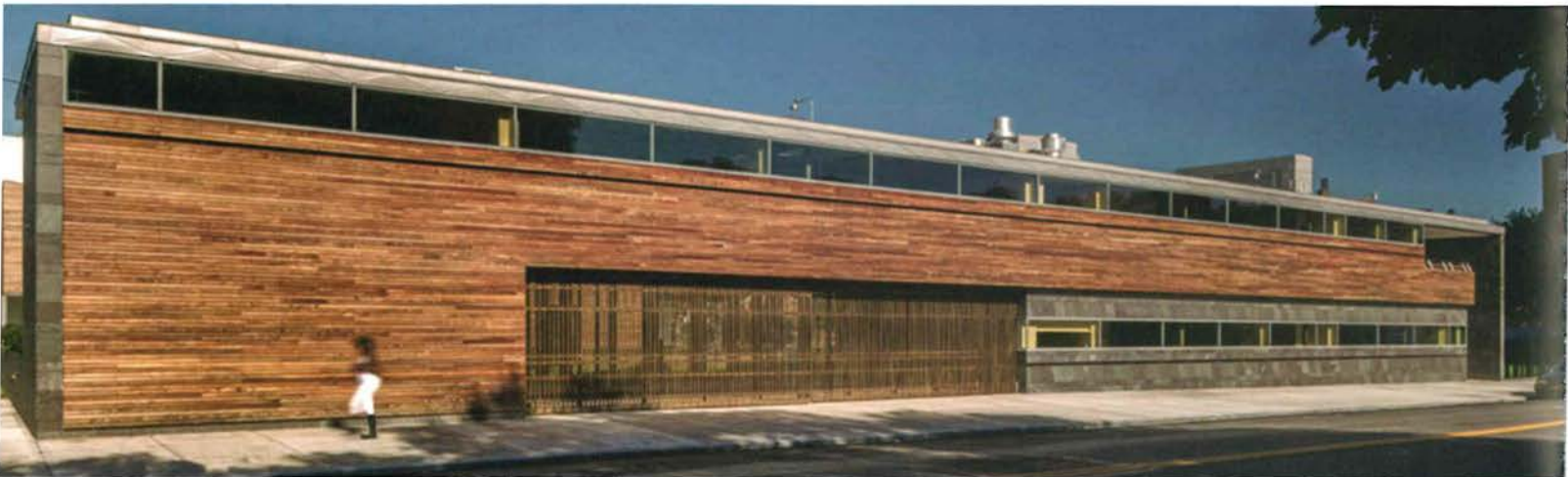
The Weeksville Heritage Center Buffalo Avenue main facade. Caples Jefferson Architects PC
