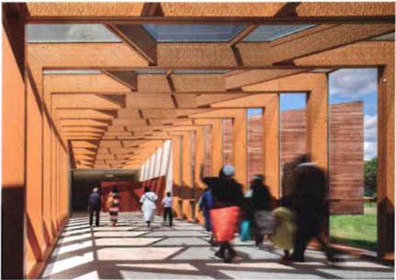
The gallery's transparent space with steel structure reminiscent of basketry bathed by textile-like shadows. Caples Jefferson Architects PC
