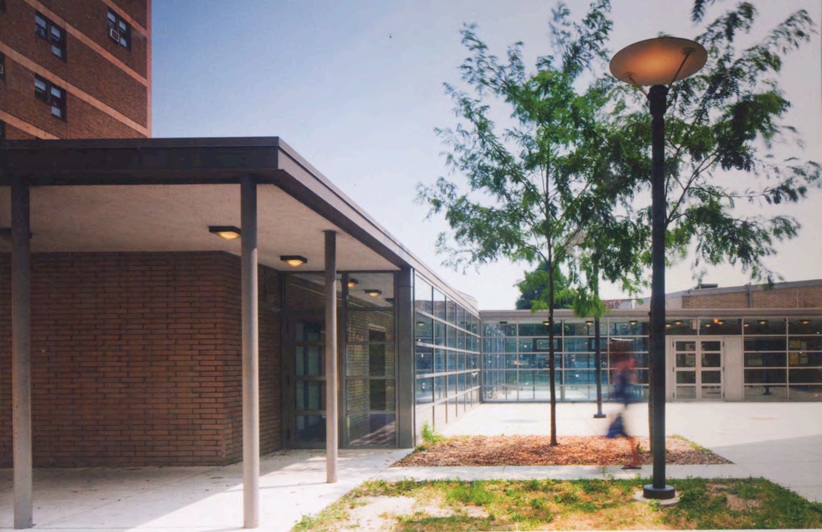
边门和老年人庭院 Side entrance and senior court
